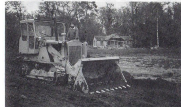
New courts under construction at Stockey Furzen.
