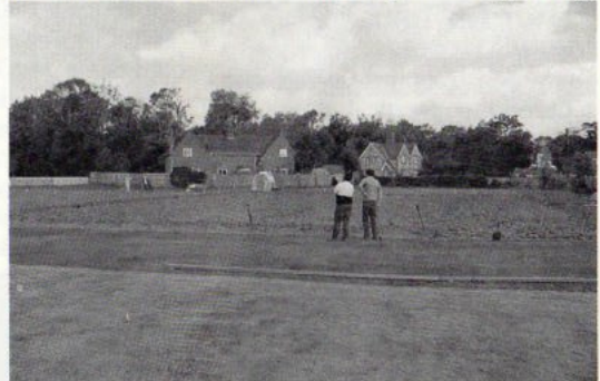
Play goes on (left) whilst the new lawns are constructed.
