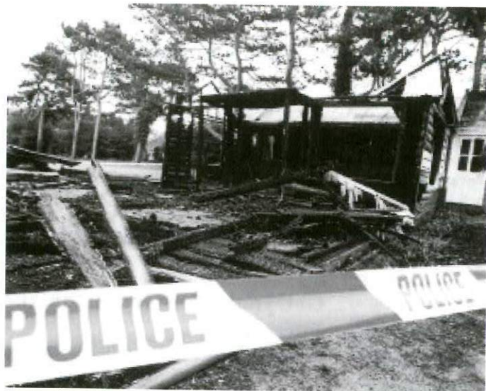
The smouldering remains of the Hunstanton pavillion. Photo courtesy of Eastern Counties Newspapers.
