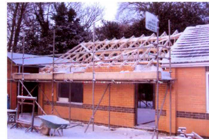
Work in progress at Cheltenham
