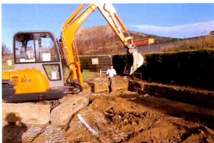
The foundations being constructed
