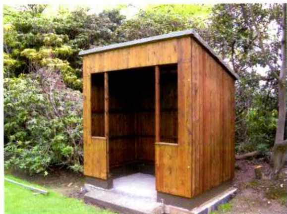
One of the completed huts at Nottingham.
