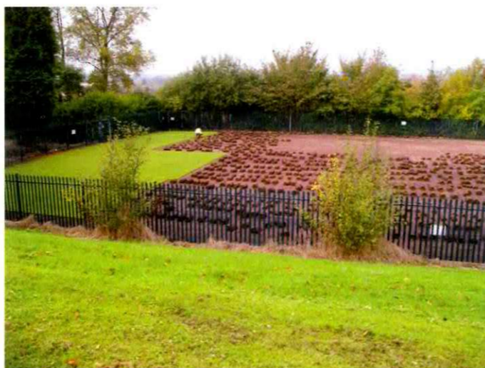
Finally the new turf is laid. Photo by Paul Rigge
