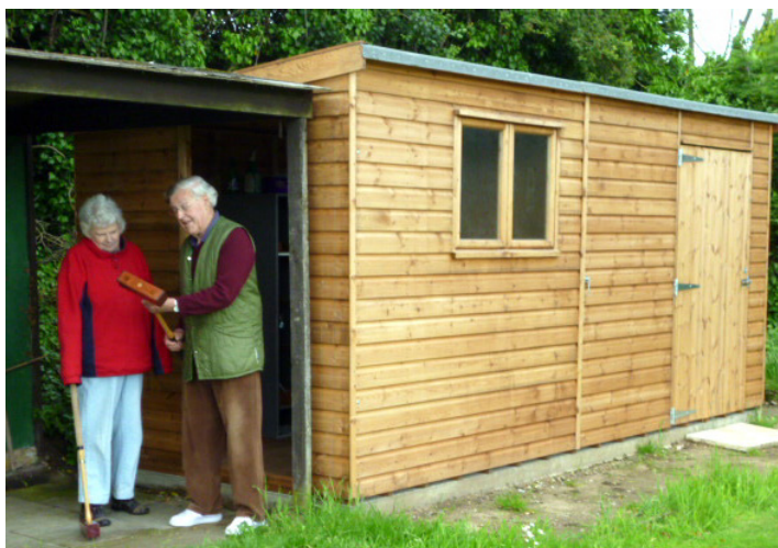
The new storage facility at Fromus CC
