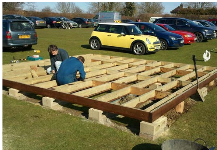
Building the base for the new pavilion
