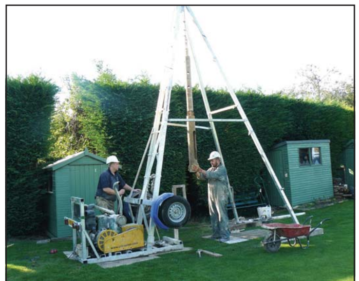
The Cruman Drilling crew ready to Break Ground
